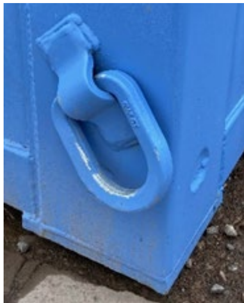
Top Lifting Positions (All SOLAR EcoLogic Welfare Units)
