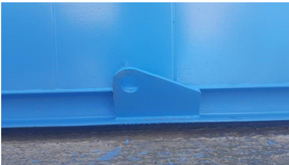
Top Lifting Positions (All EcoLogic Welfare Units)
